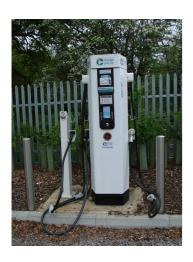
One of two new electric car chargers in Winnersh Triangle Park and Ride. These 'rapid chargers' will charge any electric car to 80% within 30 minutes, after which the machine turns off and the car must be removed. Cost 36p per KWh.
